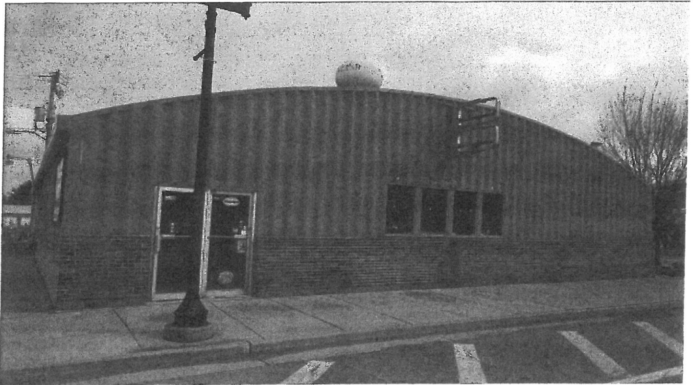
Photo #1 – South elevation.
